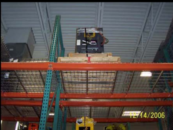
PALLETIZED LOAD, PALLET SUPPORTS MATERIAL, AND PALLET SPANS TO BOTH BEAMS
